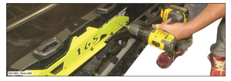
4.5 Secure bumper with 3/16" rivet [P5] in previously drilled holes as shown.
